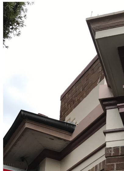
PHOTOGRAPH FROM 2018 OF THE EAVE
