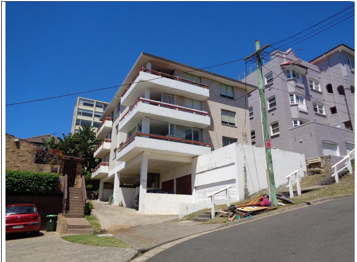
Figure 1: Subject site frontage
