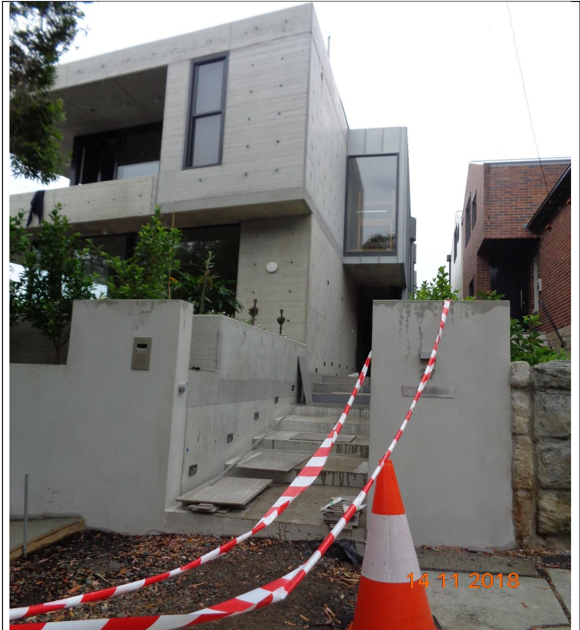
Figure 2: Pedestrian entry from Evans Street
