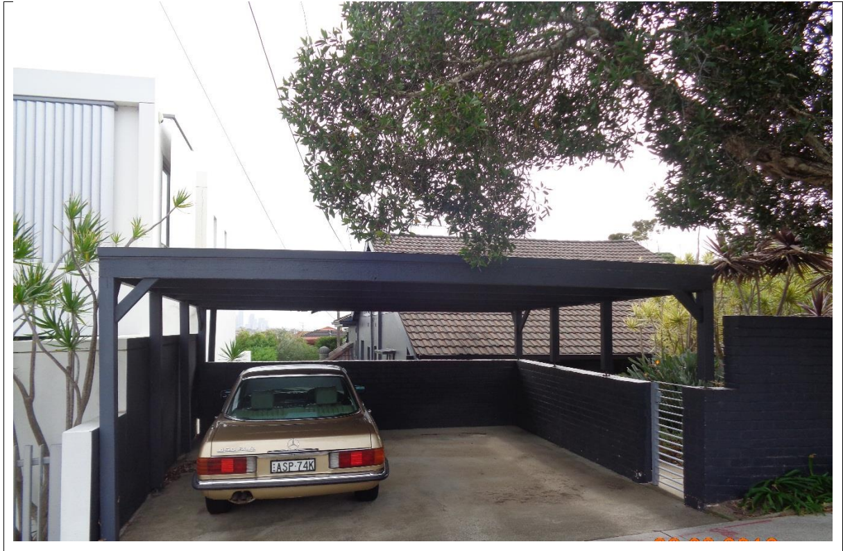
Figure 2: Existing car port on Portland Street
