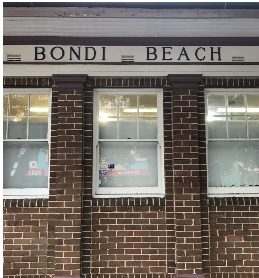
PHOTOGRAPH FROM 2018 OF HALL ST WINDOWS
