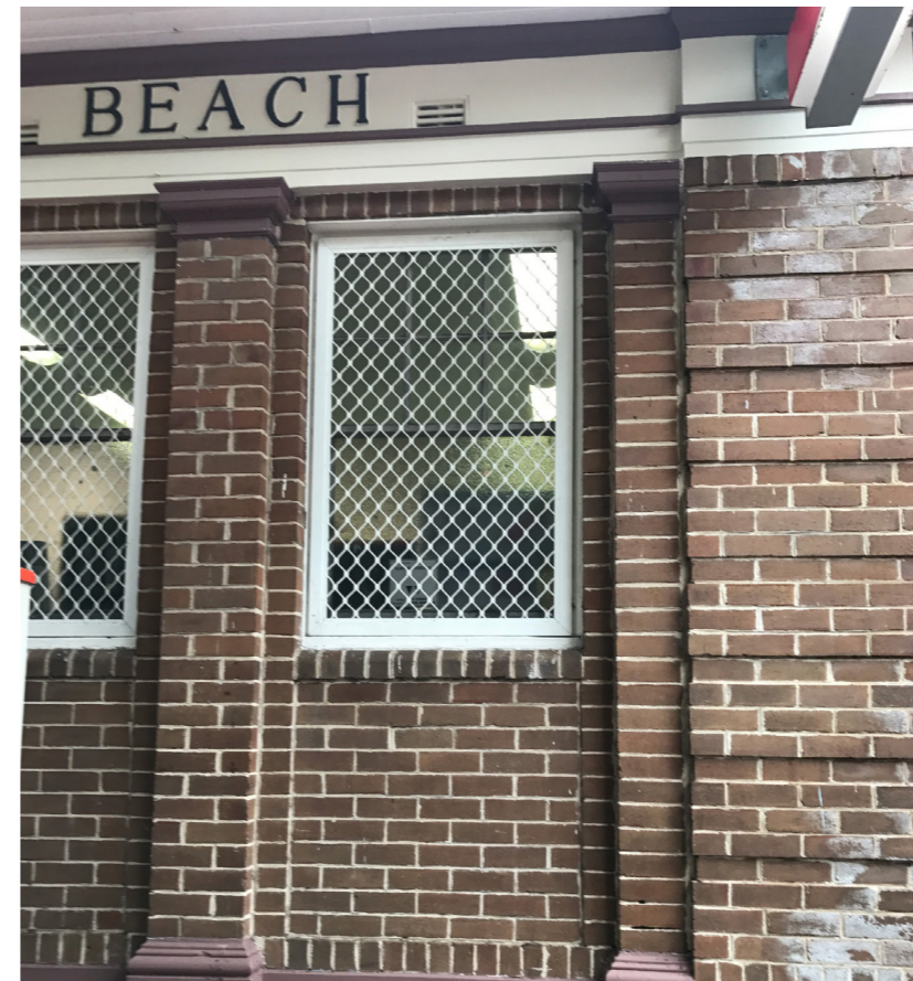
PHOTOGRAPH FROM 2018 OF JAQUES AVE WINDOWS
