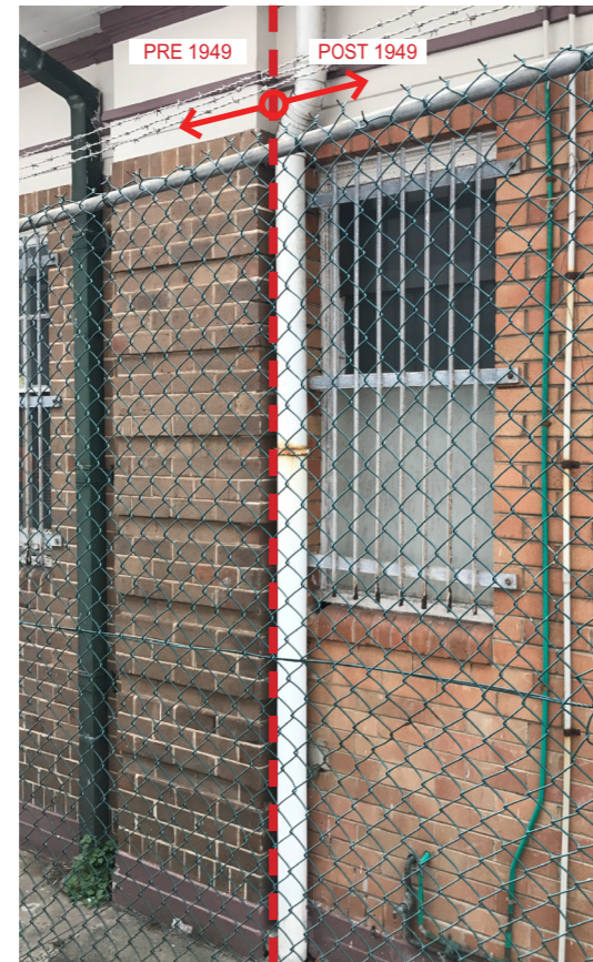
PHOTOGRAPH FROM 2018 OF POST 1949 FACADE. INCONSISTENT BRICK FINISH WITH 1934 FACADE
