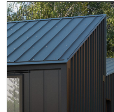
MDR & MG, RWH, DP Metal Deck Roofing: Colorbond Wide Pan Profile, Colorbond Night Sky colour + Metal Gutters, Rainwater Heads & Downpipes: Colorbond Night Sky colour
