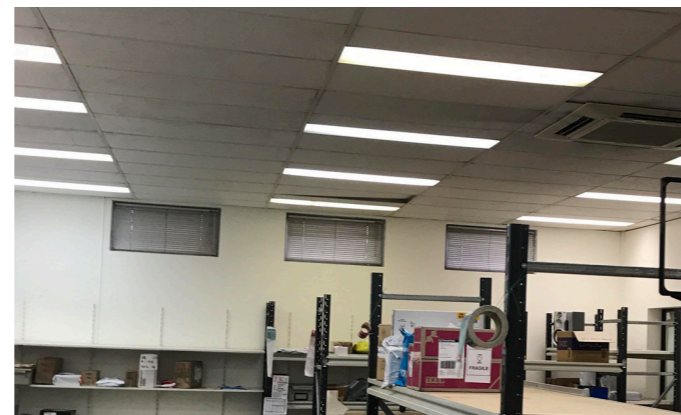
PHOTOGRAPH FROM 2018 OF POST 1949 FACADE. ONLY SMALL PORTION OF WINDOWS RETAINED
