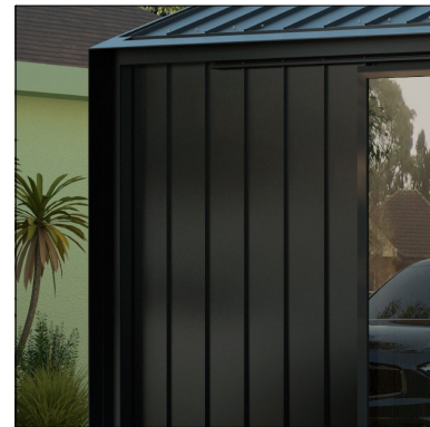
MCL & MC Metal Cladding: Colorbond Wide Pan Profile, Colorbond Night Sky colour + Metal Capping: Colorbond Night Sky colour
