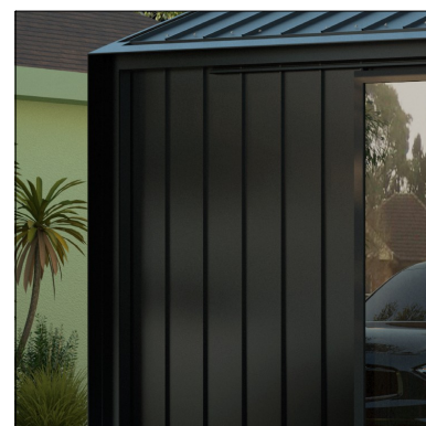
MCL & MC Metal Cladding: Colorbond Wide Pan Profile, Colorbond Night Sky colour + Metal Cappings: Colorbond Night Sky colour
