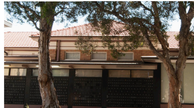
PHOTOGRAPH FROM 2018 OF POST 1949 FACADE. DAMAGED BY ADDITIONS
