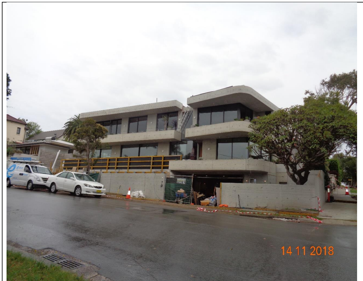
Figure 1: Site viewed from corner of Evans Street and Yanko Avenue
