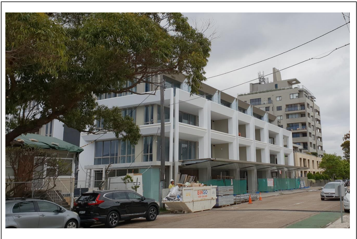
Figure 1: Subject site frontage
