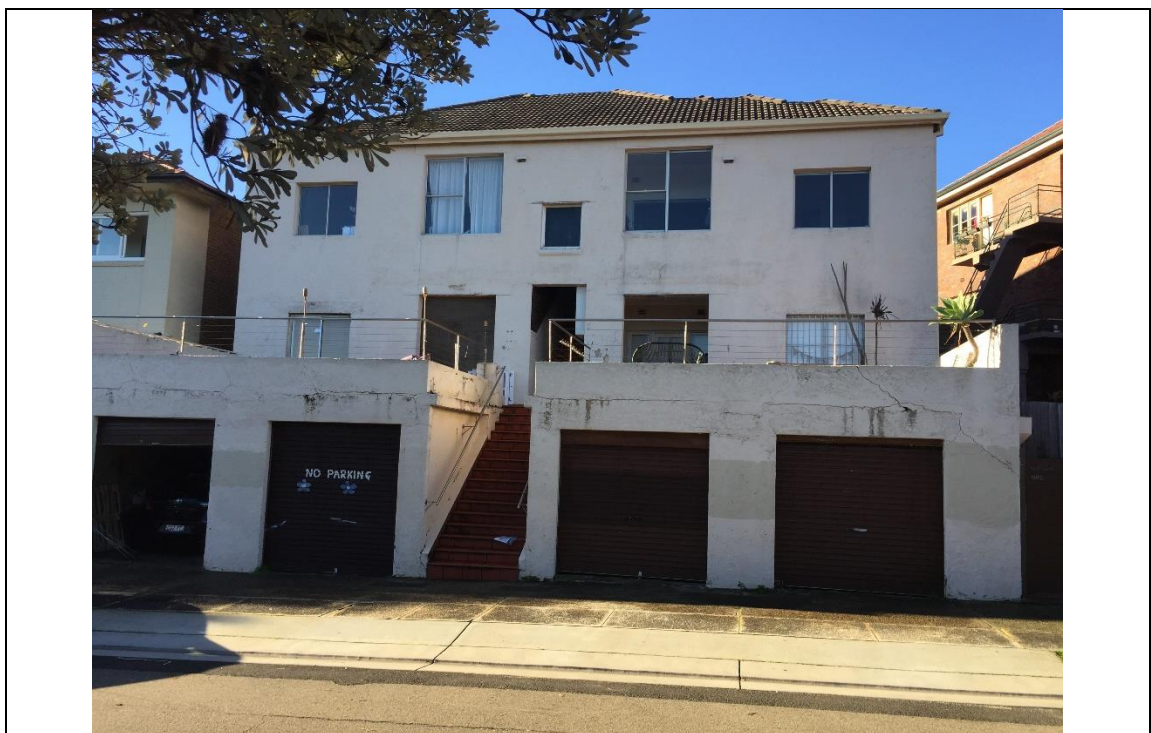
Figure 1: Subject site frontage
