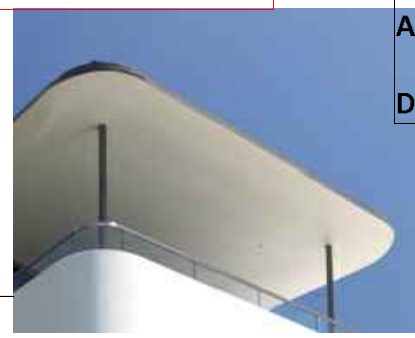
STAINED TIMBER HANDRAIL ON GLASS CEMENT RENDERED BALUSTRADE
