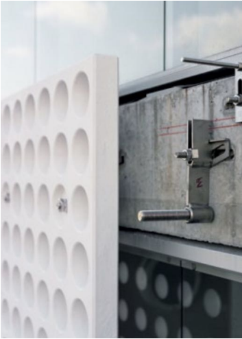
Detail of fixing to concrete slab
