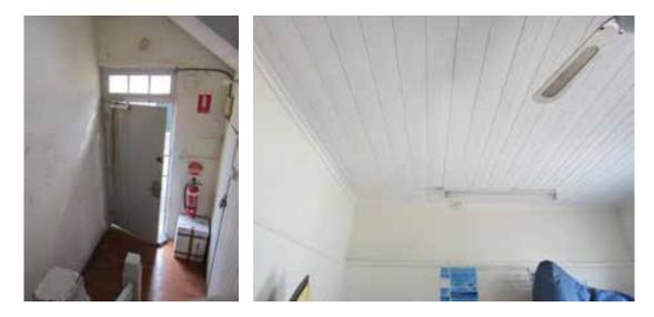
Figure 119 Ground floor vestibule associated with the stair to the former caretaker's flat (left, G45). The first floor spaces largely have timber board lined ceilings (right), although some have battened sheet linings, possibly of fibrous plaster.
