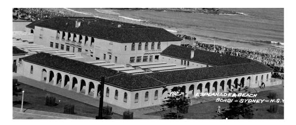
Figure 89 Part of a 1930s postcard, which clearly shows the original appearance of the western section of the two storey pavilion and the absence of a verandah attached to the single storey wing that housed the Turkish Bath. The verandah was subsequently constructed prior to the 1990s.
