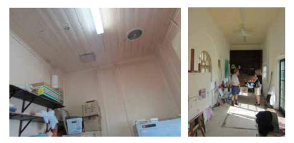
Figure 104 Although the spaces occupied by the craft studios (G4 and G5) are located in former lavatories and loggias, original fabric including timber ceiling linings, has been retained.
