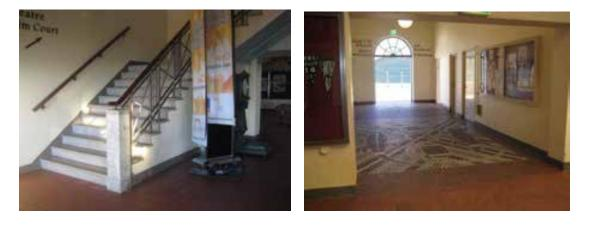
Figure 98 The original stairs leading to the first floor have marble newel posts, terrazzo stair treads and risers, wrought metal balustrades and timber handrails (left). The passage between the internal courtyards and the Bondi Pavilion's foyer, by contrast, is a modification of the original laundry (G21). It is a location of community notice boards and is enhanced by the mosaic floor featuring Aboriginal art (right).
