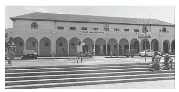
Figure 78 This 1980 photograph shows the configuration of original fenestration associated with the Turkish Bath on the western side of the principal facade and the door openings associated with retail tenancies on its eastern side. The recent arched openings in the western section of the elevation have been undertaken in a sympathetic manner, echoing the openings associated with the eastern retail spaces that already existed. Source: WL Picnumb 616.
