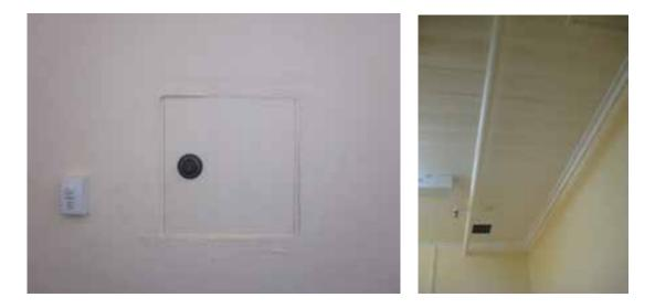
Figure 113 Intact early fabric in the eastern end of the first floor includes the safe mounted in one of the walls of the Ocean Room (left) and timber ceiling linings over the female lavatory (F7), located in spaces originally occupied by a lavatory and a storeroom. There are also early ceramic wall tiles in part of the female lavatory.
