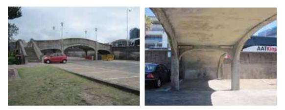
Figure 137 The form of the pedestrian bridges is typical of this period when compared to similar structures such as the bridge at Balmoral Beach. The reinforced concrete fabric of the bridges is in good condition.
