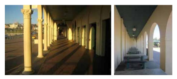
Figure 86 Views along the southern loggia (left) and western loggia with 1930s tables and benches (right). Early photographs show the floor of the southern loggia was originally concrete. The original margin beneath the columns has been retained. Loggias generally have retained timber soffit linings.
