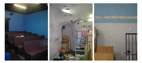
Figure 107 The fitout associated with the Marine Discovery Centre (G29) included a theatre (left) and fibreglass mouldings (centre). Wall tiles from the Turkish Bath still remain in place, though in some places concealed by later wall linings (right).
