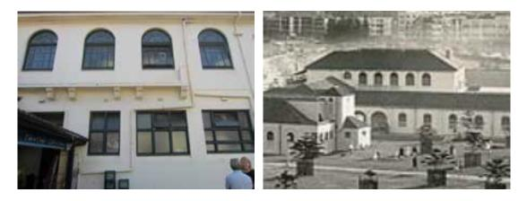
Figure 93 Evidence of a removed balconette. The absence of a sill moulding at the base of the three windows above the remnant balconette suggests that these may once have been door openings. The archival photograph indicates the presence of the balconette during the 1930s.
