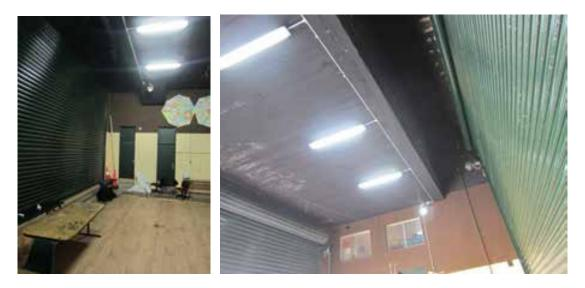
Figure 118 Stage area within the early 1930s Auditorium pavilion. The former caretaker's residence above, now used for office purposes, only extends over part of this space and has a reinforced concrete floor slab supported off a deep reinforced concrete beam.
