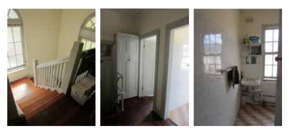
Figure 120 The first floor of the Auditorium pavilion has retained a substantial amount of original fabric including its stair (left; F28), doors, a cupboard, skirting boards and picture rails (centre; F27). However, the bathroom has been refurbished (right; F24).
