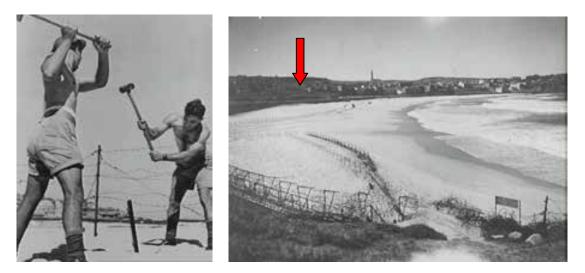
Figure 35 Installation of barbed wire on the beach, circa 1941 (left) and the completed installation, photographed on 7 July 1943. The Bondi Pavilion is indicated by the arrow; the groynes have been demolished.
