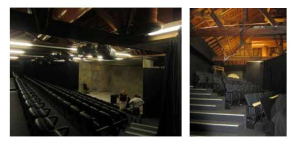
Figure 114 The Bondi Pavilion Theatre (F12), located in the original ballroom space. The Ballroom's ceiling linings were removed and the timber roof structure exposed during the conversion of the space to theatrical uses.
