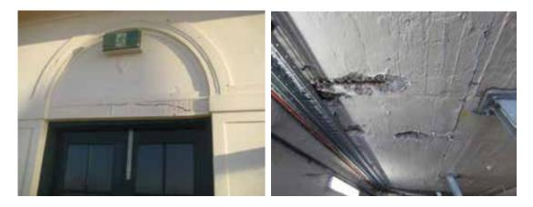
Figure 156 Cracking in rendered wall surface above a first floor door opening on the southern side of the Pavilion (left) and exposed reinforcement in the soffit of a groyne tunnel (right).
