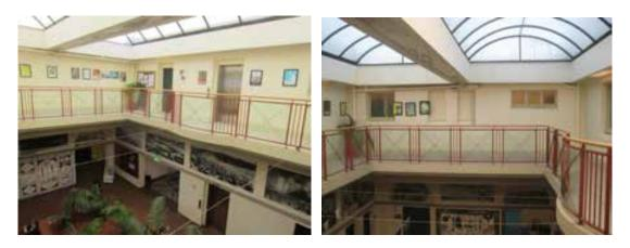
Figure 109 Upper level of the Atrium (F10), originally a light court and modified by the construction of a perimeter mezzanine and enclosed by translucent vaults.
