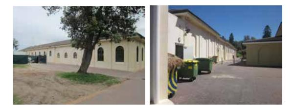
Figure 85 The western side of the Pavilion complex has been subjected to a relatively high level of change, including the enclosure of the pair of loggias and modifications to original window openings. Those on the beach side of the building have been blocked up or covered over).
