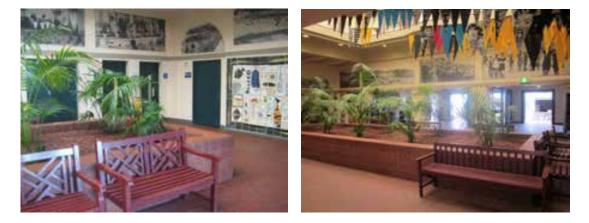
Figure 99 The former bathing costume/towel hire area and light well have been modified and opened up on its eastern side to become an atrium. The well-intentioned brick planter is an inappropriate element within the space. Interpretive photographs have been mounted around the space. Quarry tiles covering the floor are not original.
