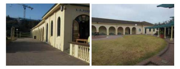
Figure 82 Looking north along the western facade. The balustrade has been modified to provide access to the tenancy space that now occupies the shower room (left). The western facade incorporates a secluded loggia (right).
