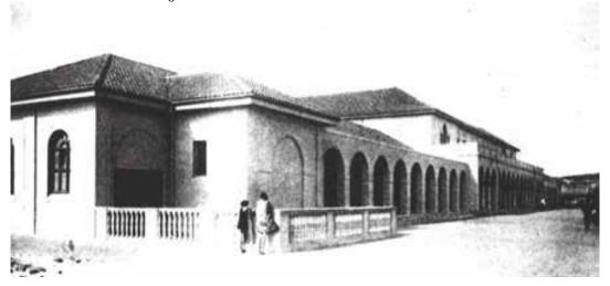
Figure 81 Circa 1930 photograph looking north along the principal facade of the Pavilion, showing the low balustrade that defined the entry to spaces then occupied by women's showers. The door opening has been modified and the blind arched panel formed into a door opening. Source: reproduced in *The Home*, April 1930.
