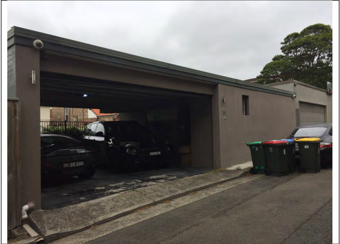
Figure 2: Existing garage/storage viewed from York Lane at the rear
