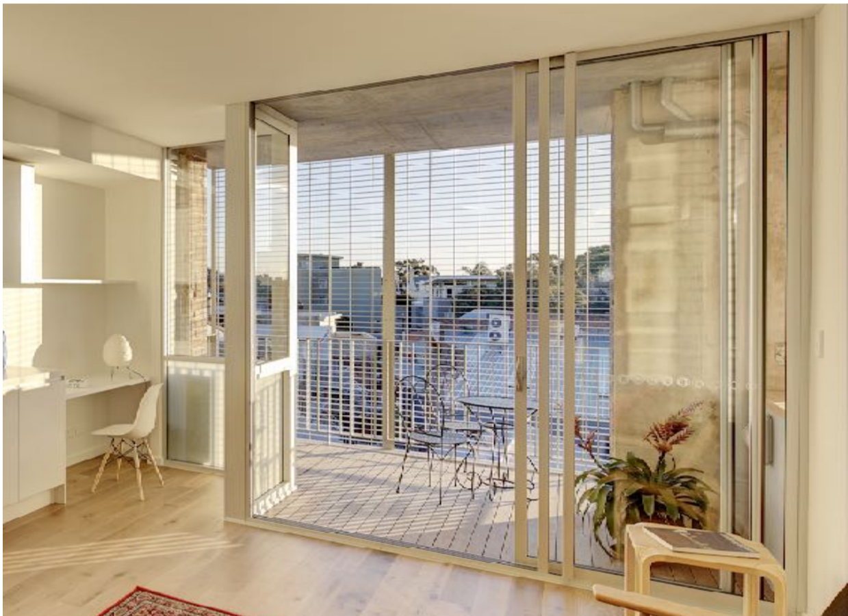
AFW/ AFD - Aluminium framed windows / doors * upper levels in MR dormer to be powdercoated to match MR ** windows within brickwork to be white powdercoated
