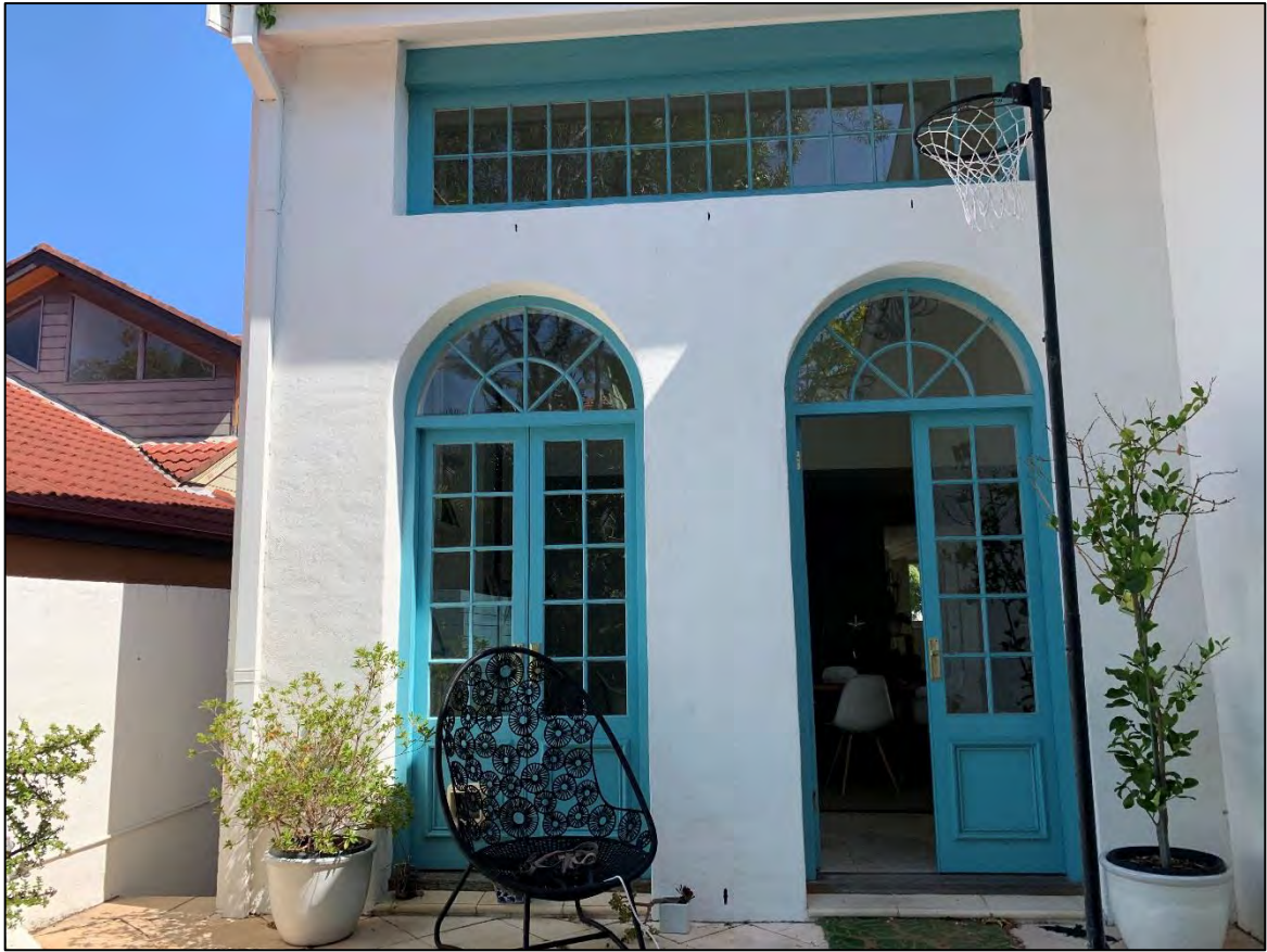
Figure 2: Existing front entrance to dwelling.
