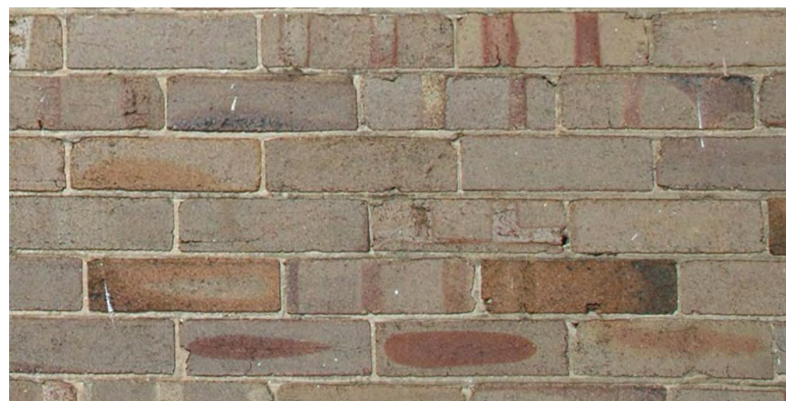
BRK1 - D\Dry Pressed Old Sydney Common Brick to match existing brick
