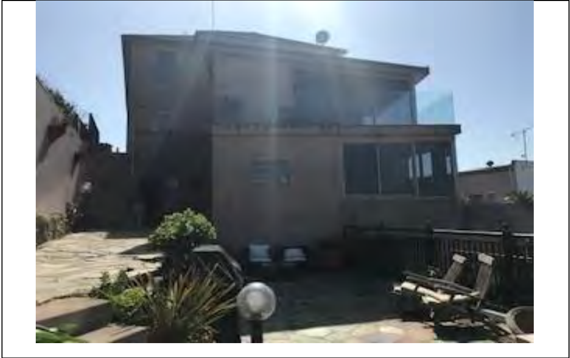
Figure 2: Rear of building
