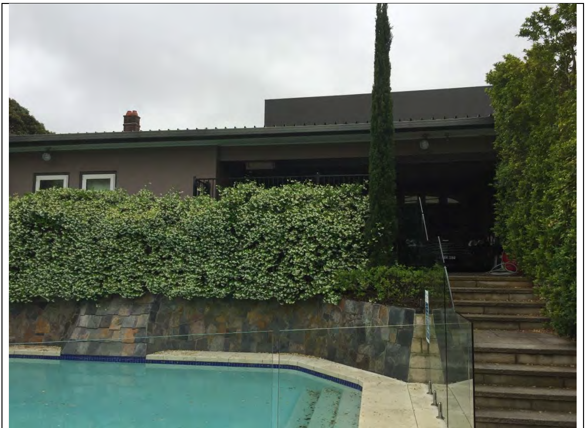
Figure 1: Rear of the site looking from the dwelling toward the existing rear garage/storage
