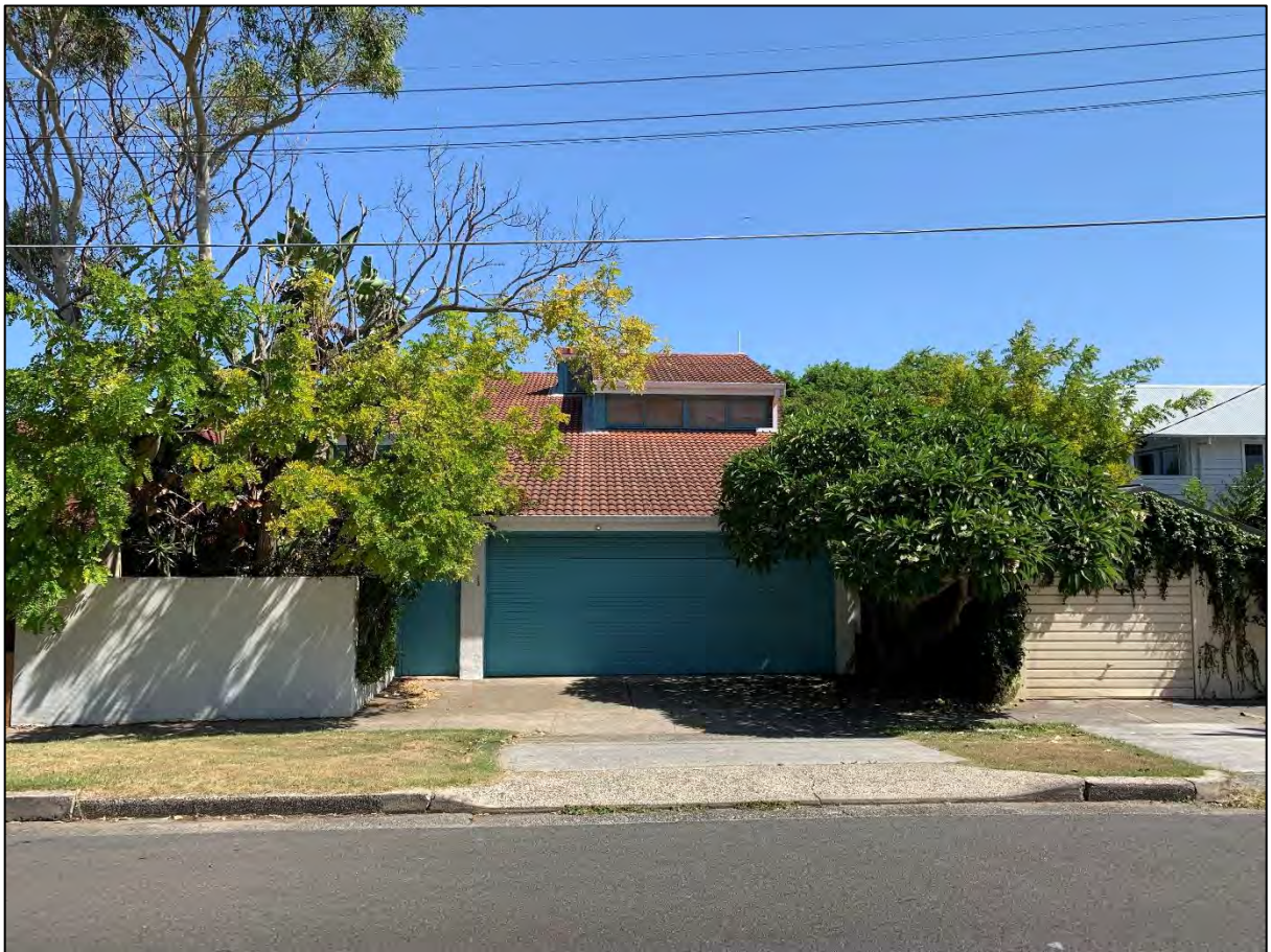
Figure 1: Site viewed from Darling Street.
