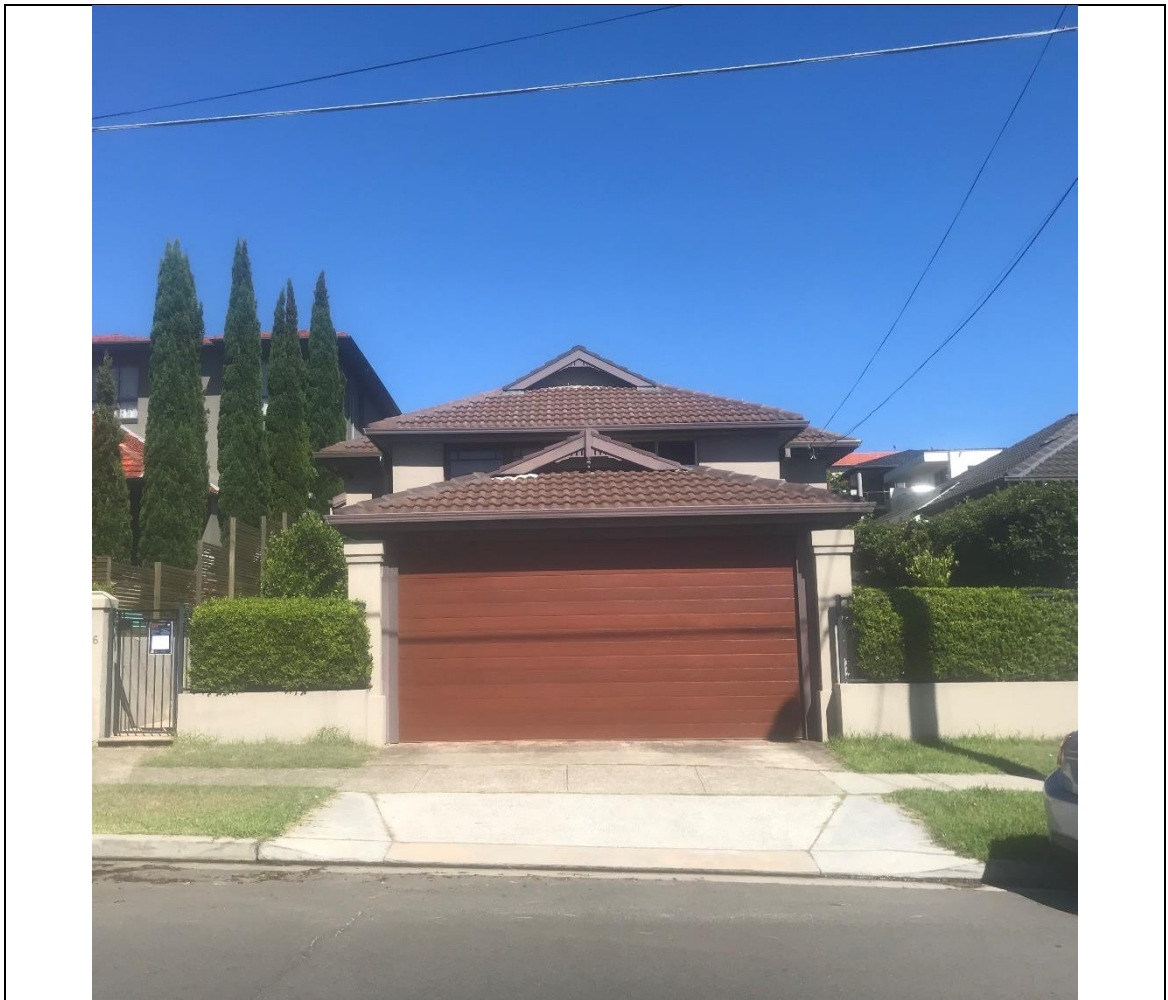
Figure 1: Site viewed from Military Road
