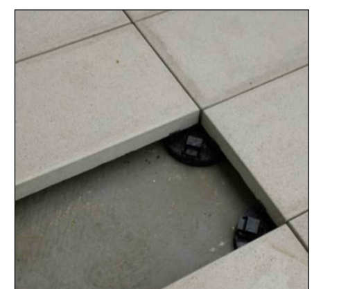
ROOF DECK PAVING
