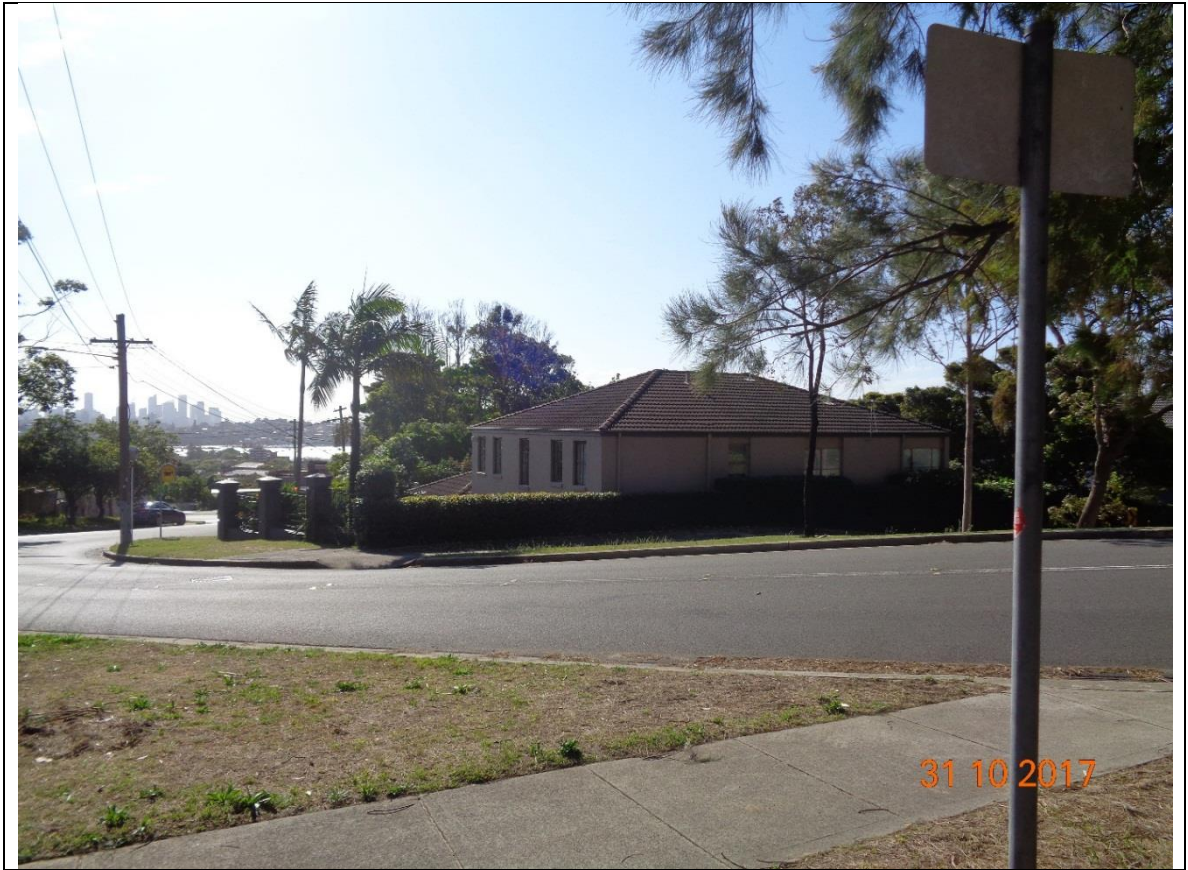
Figure 2: Site viewed from the east (side elevation with Gilbert Street)
