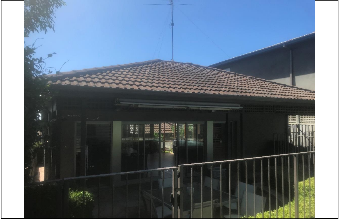
Figure 2: Existing rear elevation of the site
