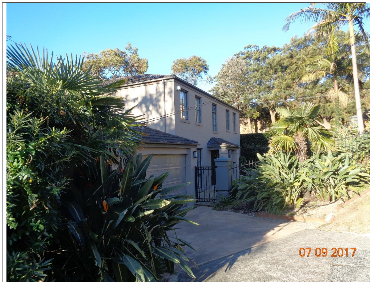
Figure 1: Site viewed from Victory Street
