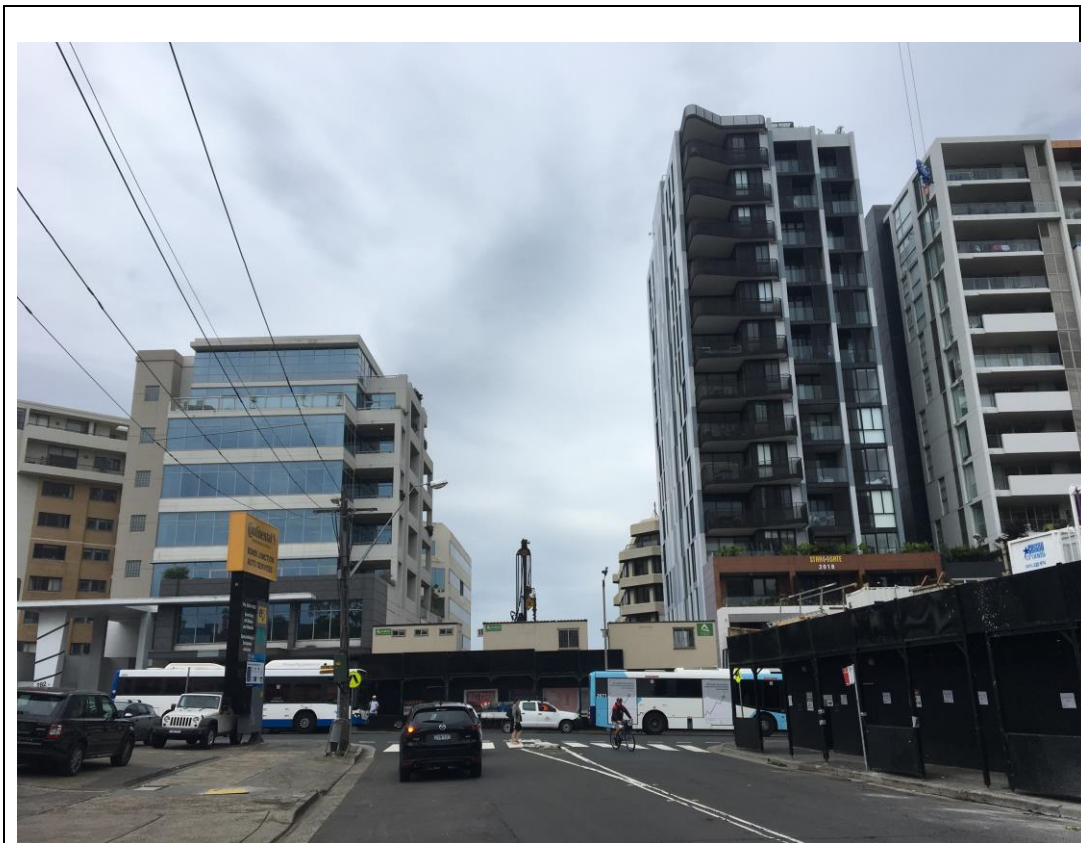
Figure 1: Subject site frontage
