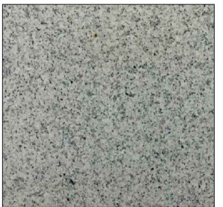
THROUGH SITE LINK & LOBBY TILING
