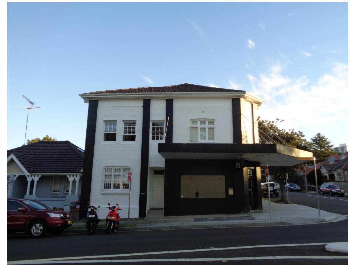
Figure 1: Site viewed from Lamrock Avenue
