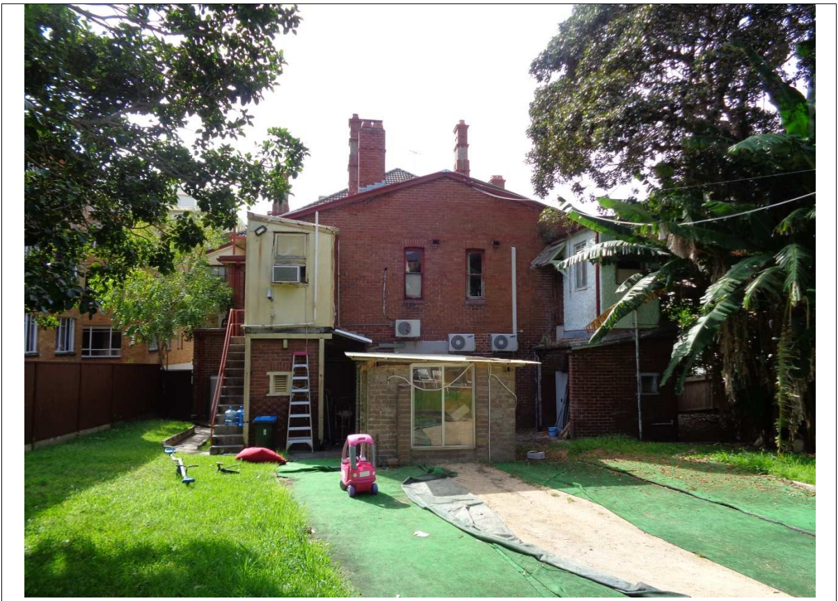
Figure 3: Rear elevation of the building
