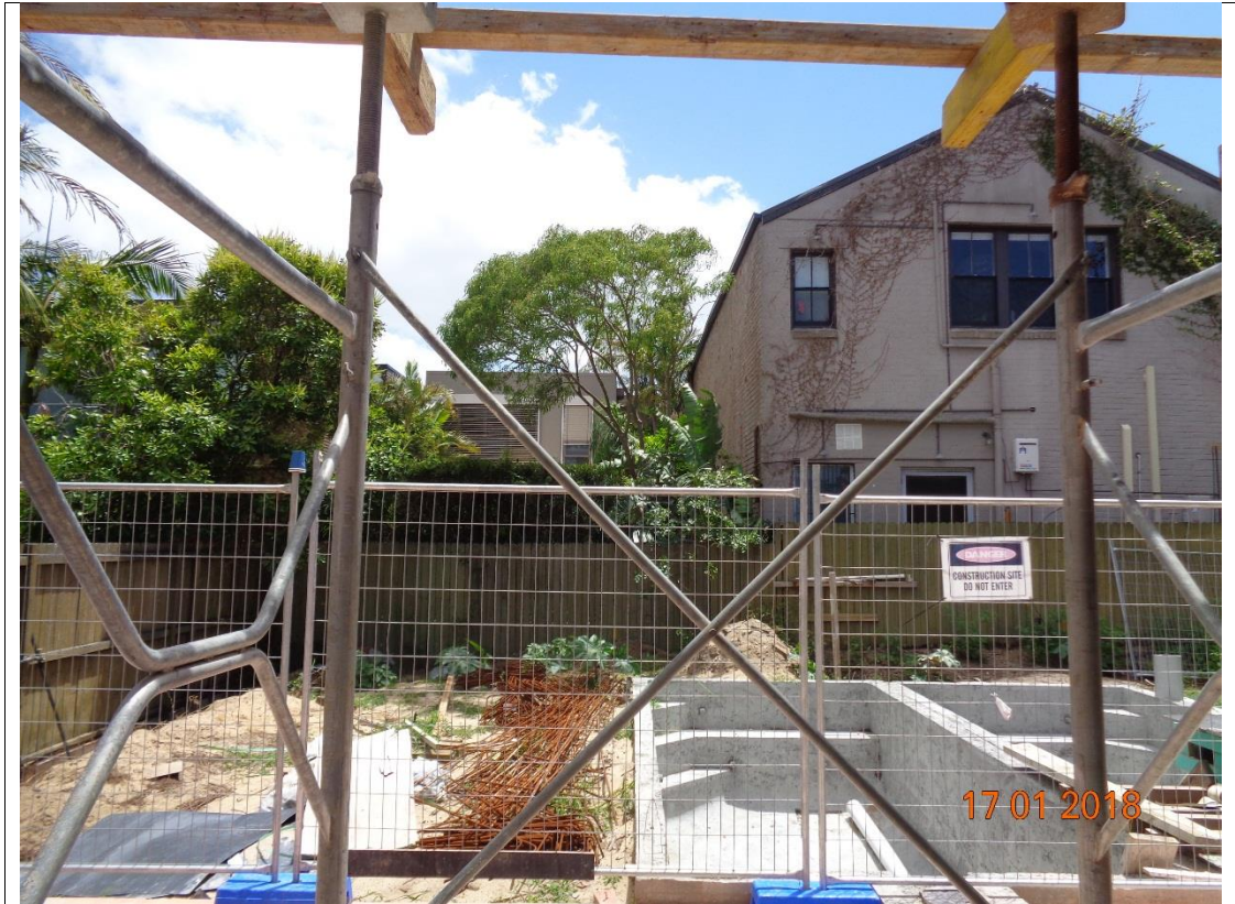
Figure 4: Site viewed from the rear also showing adjoining property to the rear at No.5 Roberts Street
