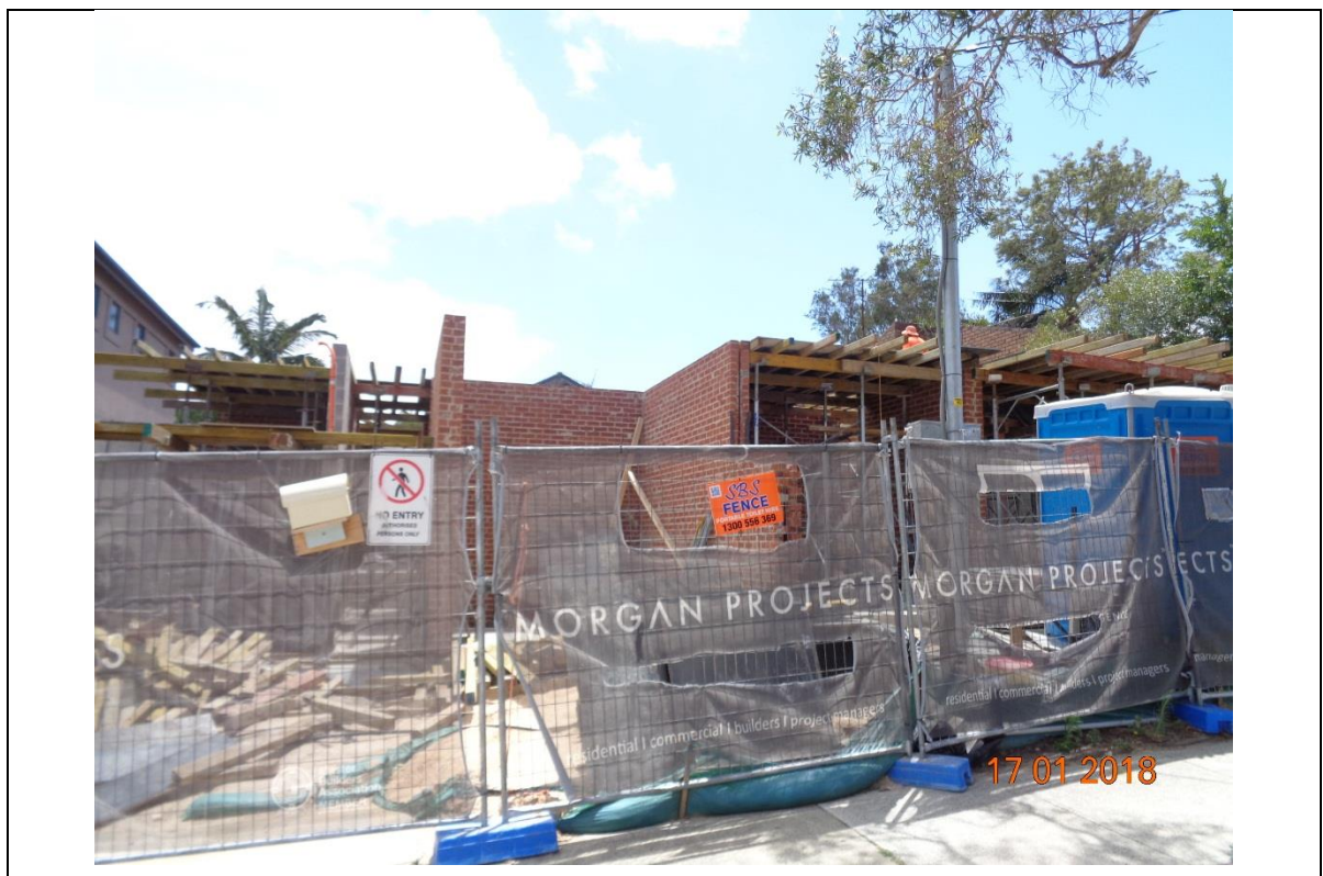
Figure 1: Subject site frontage
