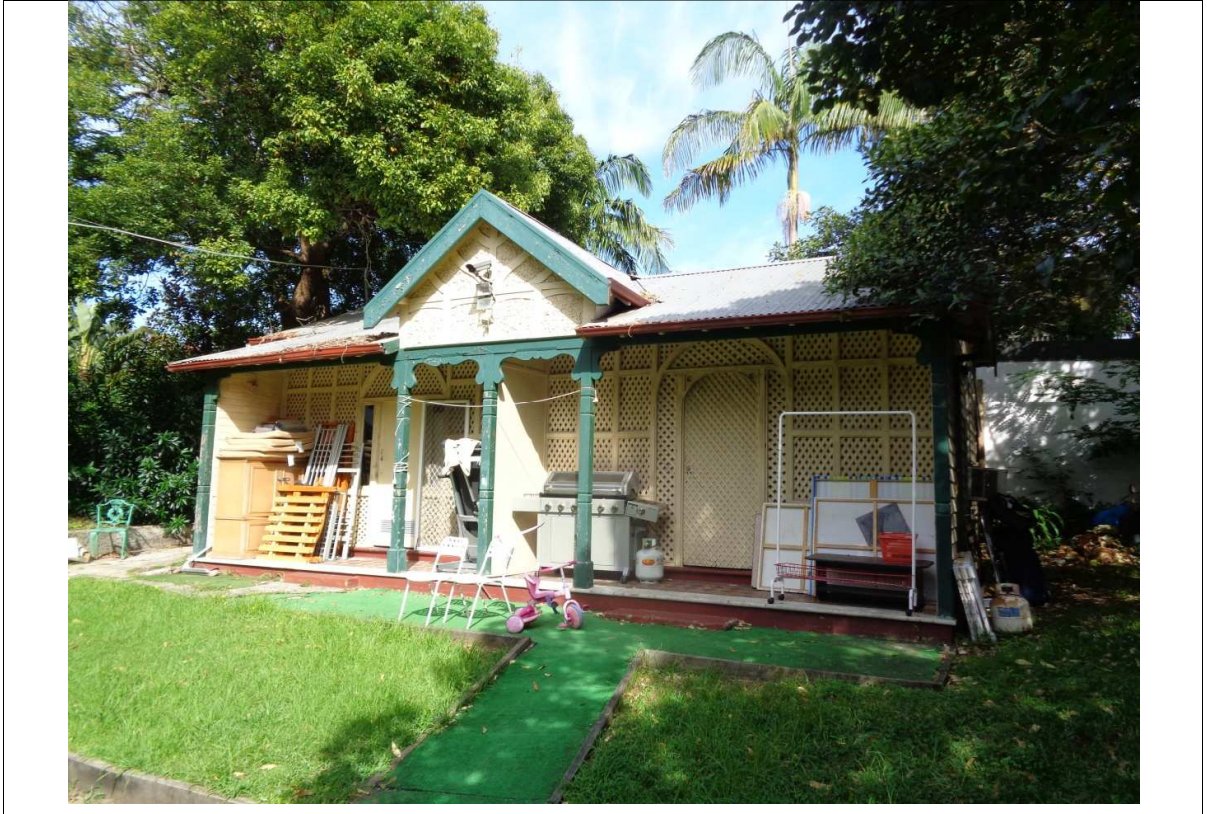
Figure 4: Outbuilding within the rear setback
