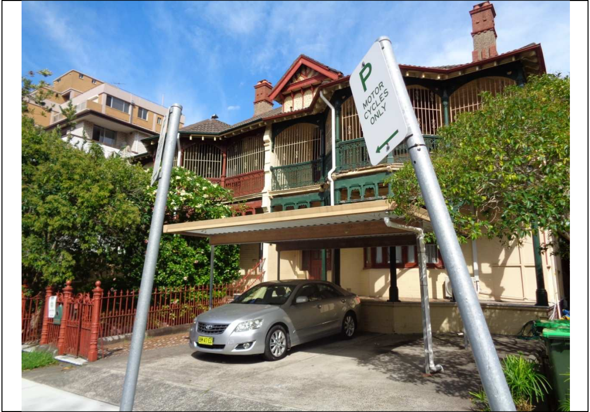
Figure 2: Subject site frontage
